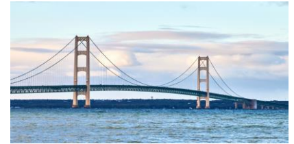
About 42,000 miles of wire make up the main suspension cables of the Mackinac Bridge in Michigan.
